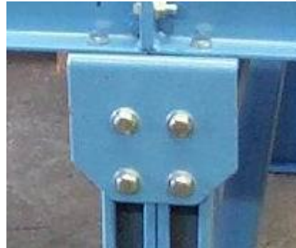
HD SUPPORT MOUNTED ON JOINT
