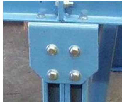
HD SUPPORT MOUNTED ON JOINT
